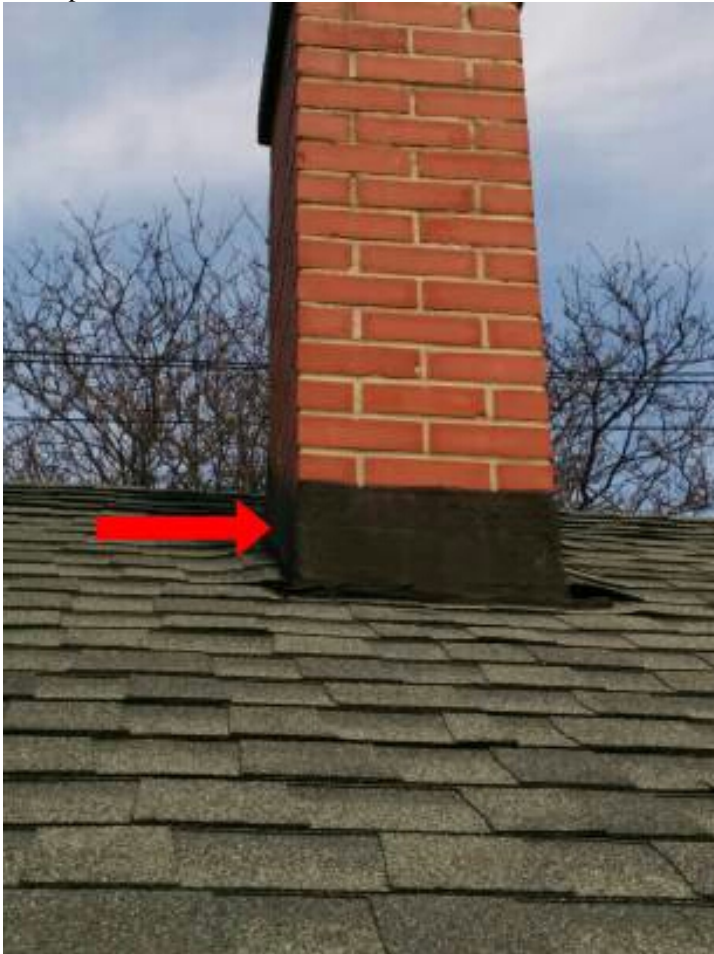
Chimney flashing covered with roofing cement not visible.
