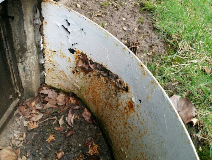
Rusting of window wells repair/replace as needed
