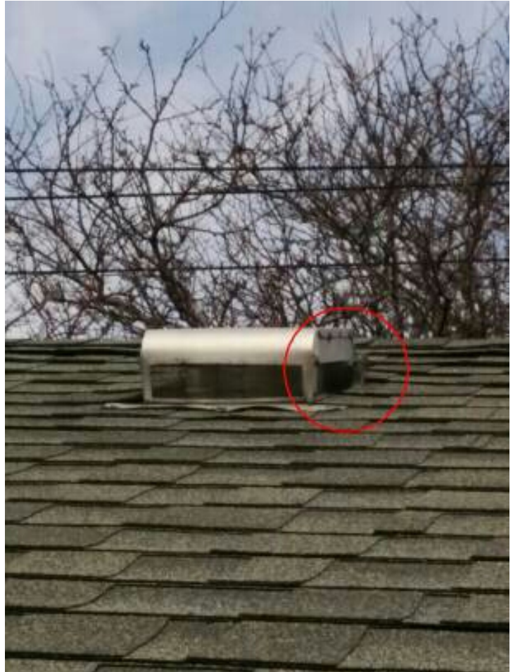
Damaged screen on roof vent recommend replacing screen to prevent pests from entering attic
