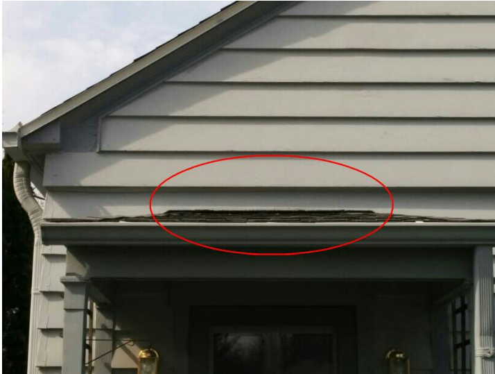
Missing wall to roof flashing recommend installing one to prevent water penetration into home.
