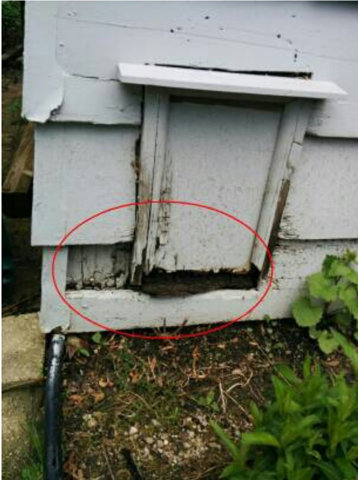
Areas of siding on garage are damaged recommend repair/replacing damaged areas as needed.
