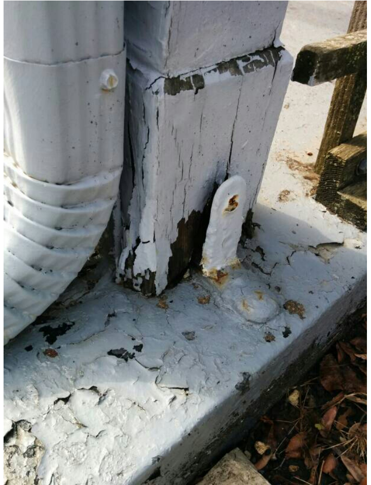
Wood rot on support pier on front porch recommend replacing damaged wood.
